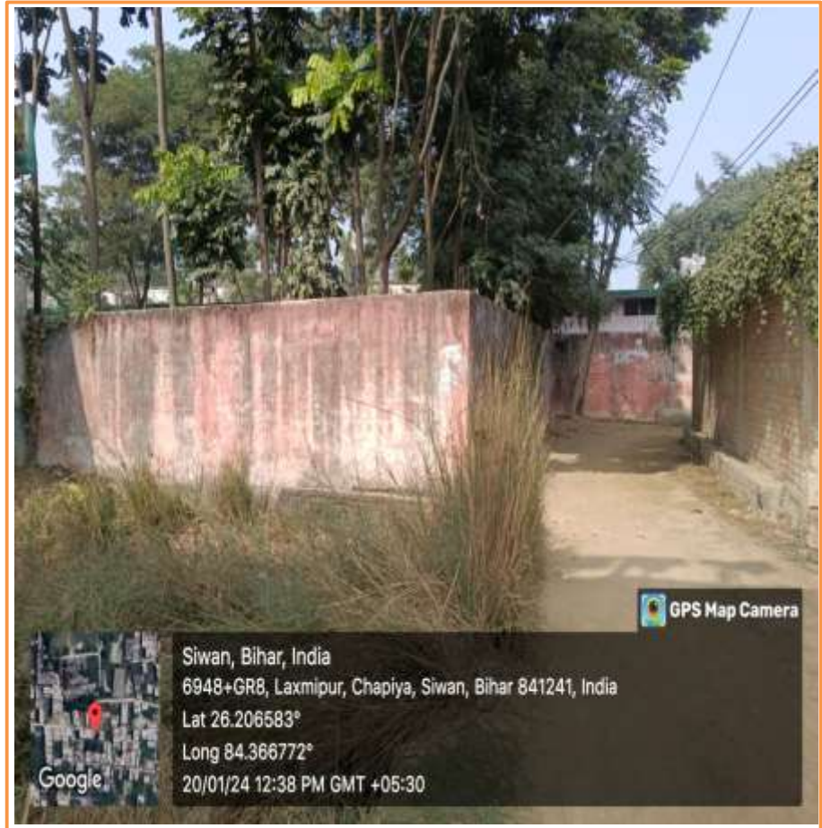
BOUNDARY 2 (OUT SIDE PHOTOGRAPH)
